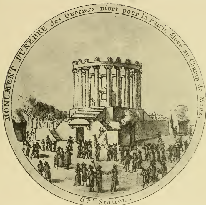
Plate 155. A representation of the sixth stage of the Fête to Unity and Indivisibility. The temple is in honour of the dead warriors.
